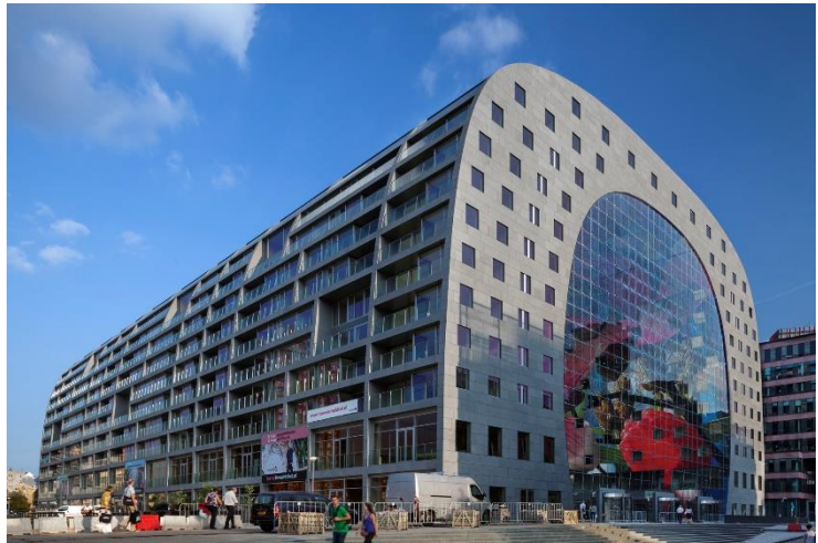
Figure 18 the Rotterdam market hall
