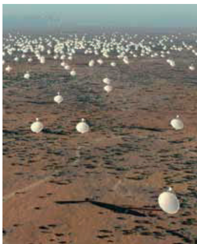
The SKA will consist of an inner core and outer stations arranged in a log-spiral pattern and extending to distances of up to at least 3,000 km (Copyright: SPDO).
