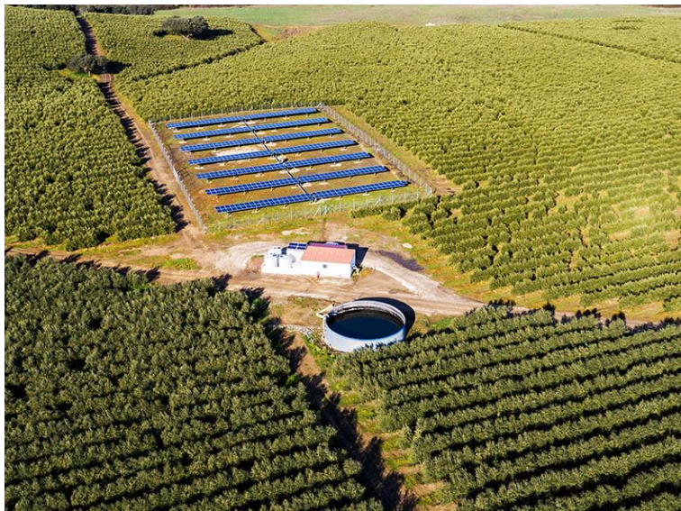
140 kWp – PV/Diesel - Drip Agro-industry Portugal
