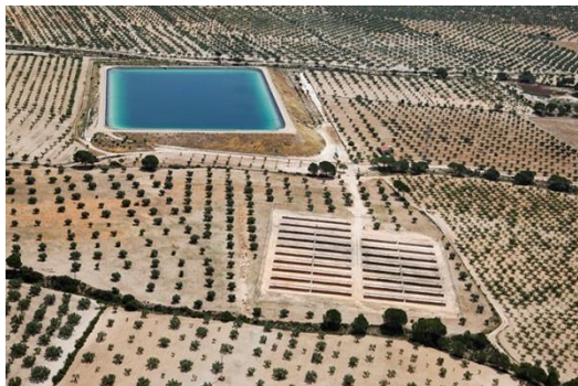
360 kWp – Water Pool Irrigator Community Spain
